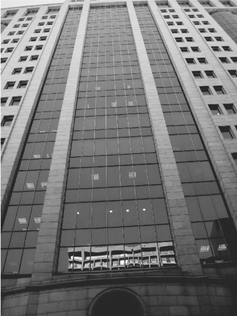
Figure 1.2. Anglo Platinum headquarters, Johannesburg. Author’s photograph.
